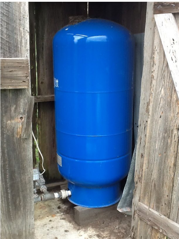
Booster Pump Pressure Tank
