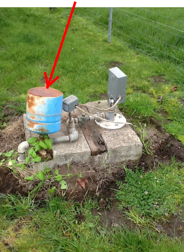
Well Pump Pressure Tank
